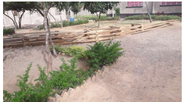
Roo truses being constructed
